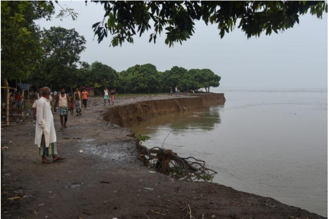
Image No 7 : Bank Erosion , Samsenguange Block, Murshidabad.
